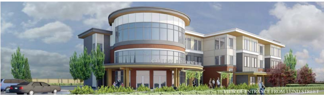
VIEW OF ENTRANCE FROM 132ND STREET
