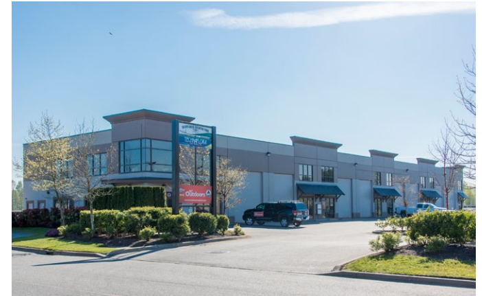
Retail/Office at Silver Creek Business Park
